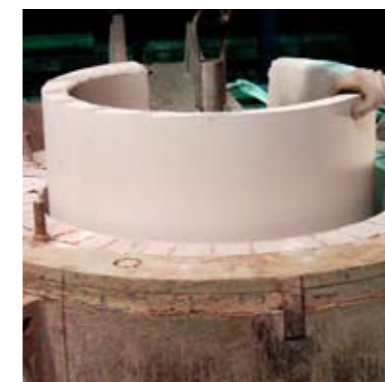
Then insert the DORIT prefabricated crucible by using a lifting device.
